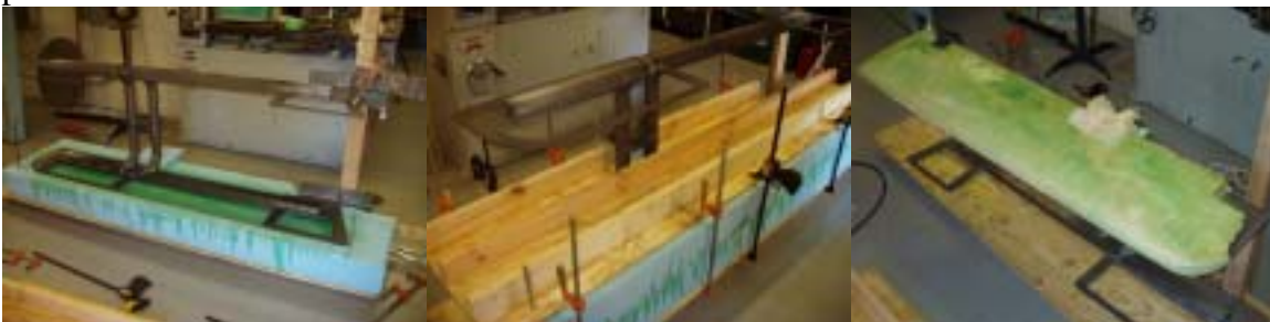
Figure 12- The first pontoon being cast.
