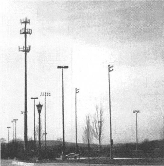
Figure 9.21 Cellular Telephone Antenna
