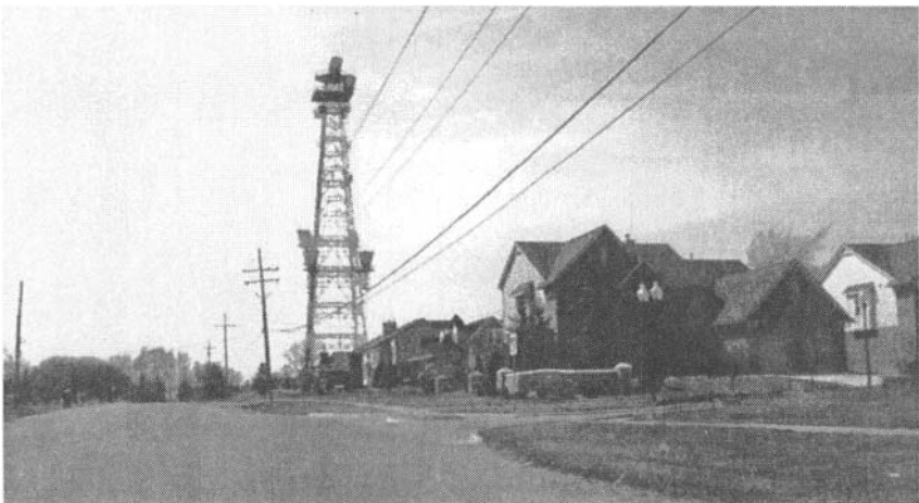
Figure 9.22 Microwave Relay Tower
