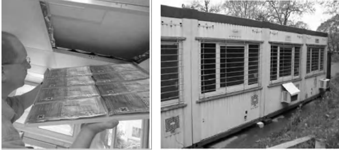
Fig. 9.18. Left: Installation of Dörkens DELTA ® -COOL 24 on top of a suspended ceiling. Right: Containers equipped with DELTA ® -COOL 24 for a field study performed in 2003 (pictures: Dörken)
