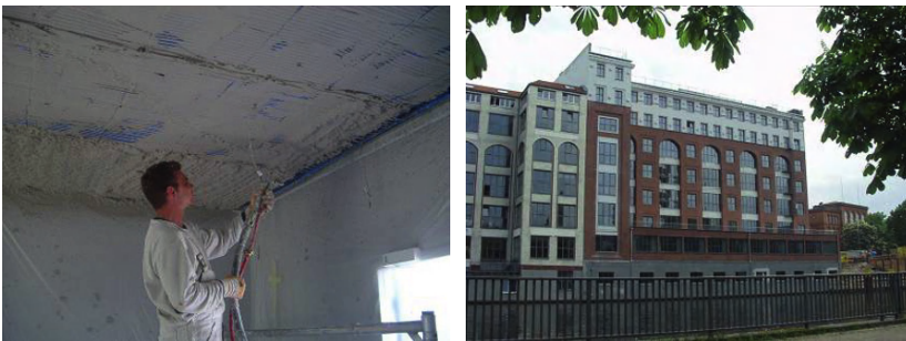
Fig. 9.32. Installation of 1100 m 2 plaster maxit clima ® on capillary sheets (picture: FhG-ISE) in a building in Berlin (picture: M. Schmidt).
