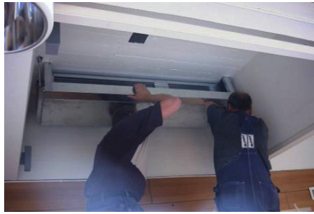
Fig. 9.30. Cooling and ventilation system integrated into the ventilation channel, developed by the company Climator (picture: Climator)
