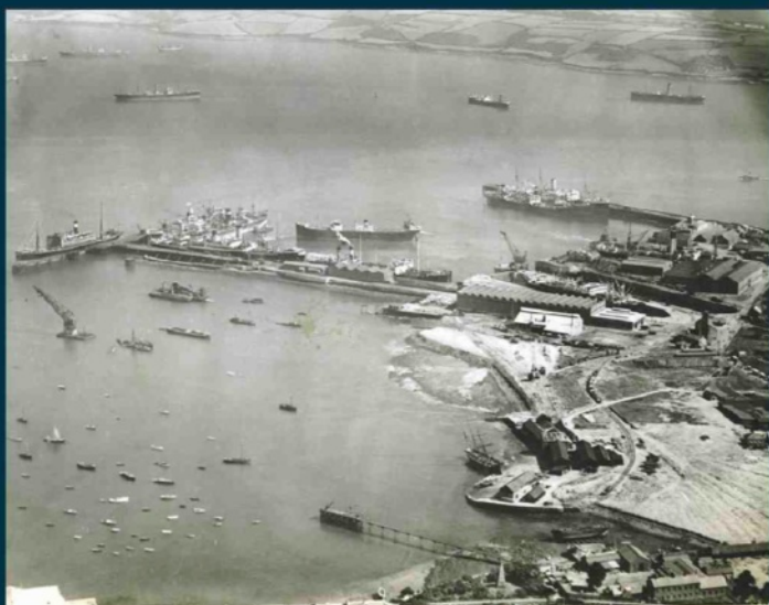
ABOVE: An aerial view of Falmouth Docks and the Submarine Pier taken in 1928, with the dredger Briton and floating crane prominent. The Submarine Pier, built by the Falmouth Volunteer Division of Submarine Miners (Royal Engineers), was part of the coastal defences and was never intended for use by submarines. The dredger was used to ensure the channels and dock area were maintained, and the port was regularly dredged until the late 1970s. In the foreground is the Bar area, which comprised boatbuilding slipways and sheds and was redeveloped in the 1980s into waterside apartments and latterly the excellent National Maritime Museum.
