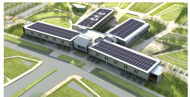
Fig. 9 Example of PV Installation at Ohlone College, Newark Center, Newark, CA: 450 kW, 38,000 ft 2 (Esberg 2010)
