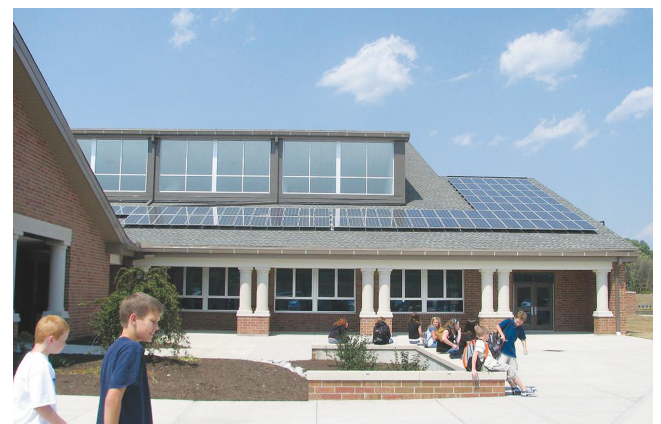
Fig. 10 Example of PV Installation at Twenhofel Middle School, Independence, KY: 22 kW (Seibert 2010)
