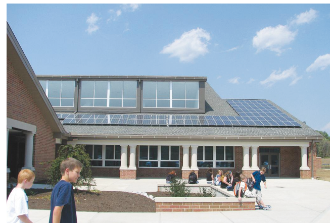
Fig. 10 Example of PV Installation at Twenhofel Middle School, Independence, KY: 22 kW (Seibert 2010)
