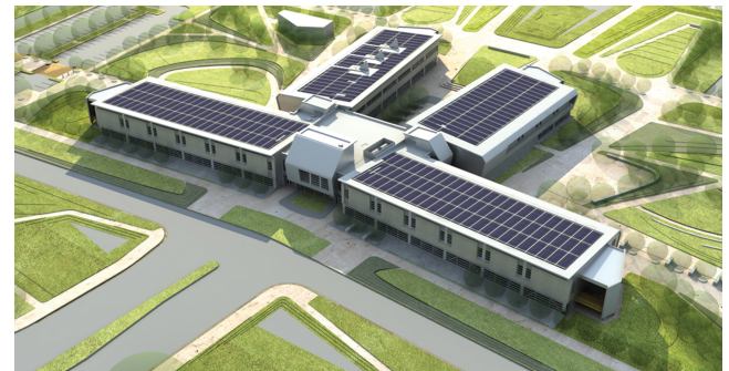
Fig. 9 Example of PV Installation at Ohlone College, Newark Center, Newark, CA: 450 kW, 3530 m 2 (Esberg 2010)
