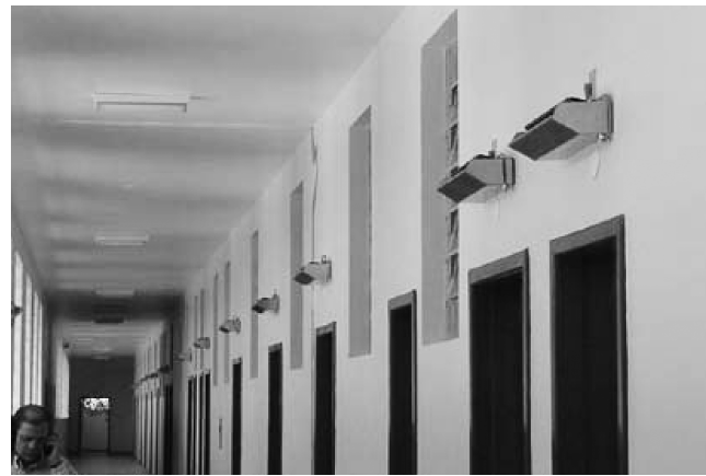
Fig. 8 Upper-Air UVC Devices In A Naturally Ventilated Corridor of TB Facility in Brazil (Centers for Disease Control and Prevention)
