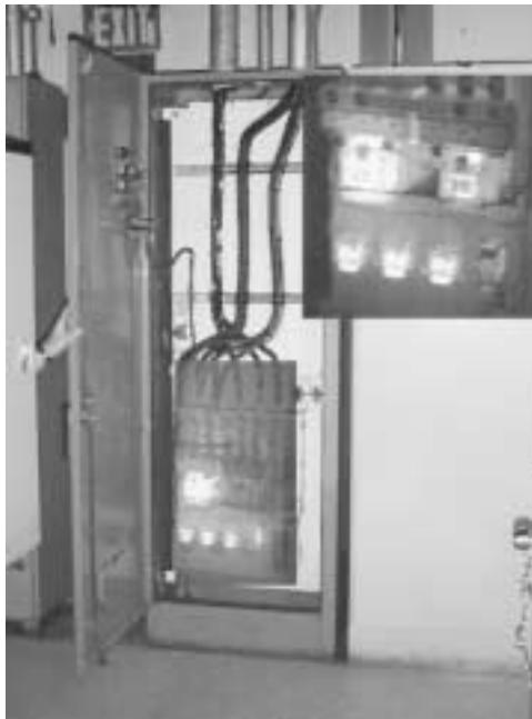
FIGURE 9. Infrared thermography of automatic transfer switches of emergency diesel generator. Hot spots appear bright in thermogram.
