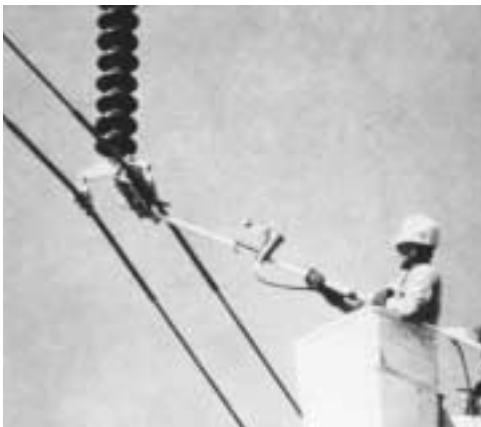
FIGURE 34. Lineman using hot line X-ray equipment. 36
