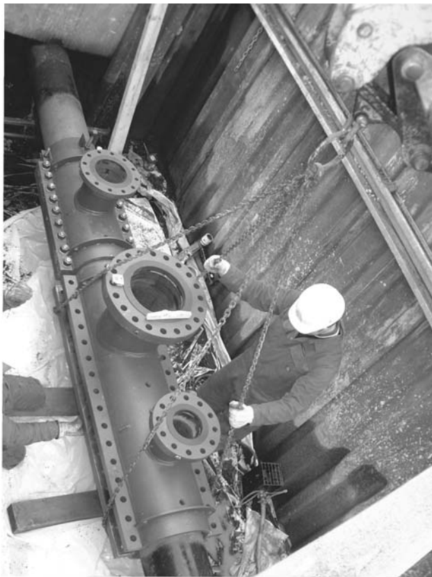
Figure 8.4 Grouted ™ tee connection
