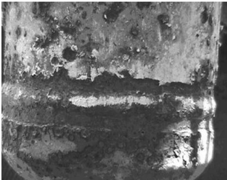
Fig. 4-64—Oxidation of the O.D. of a carbon steel furnace transfer line.
