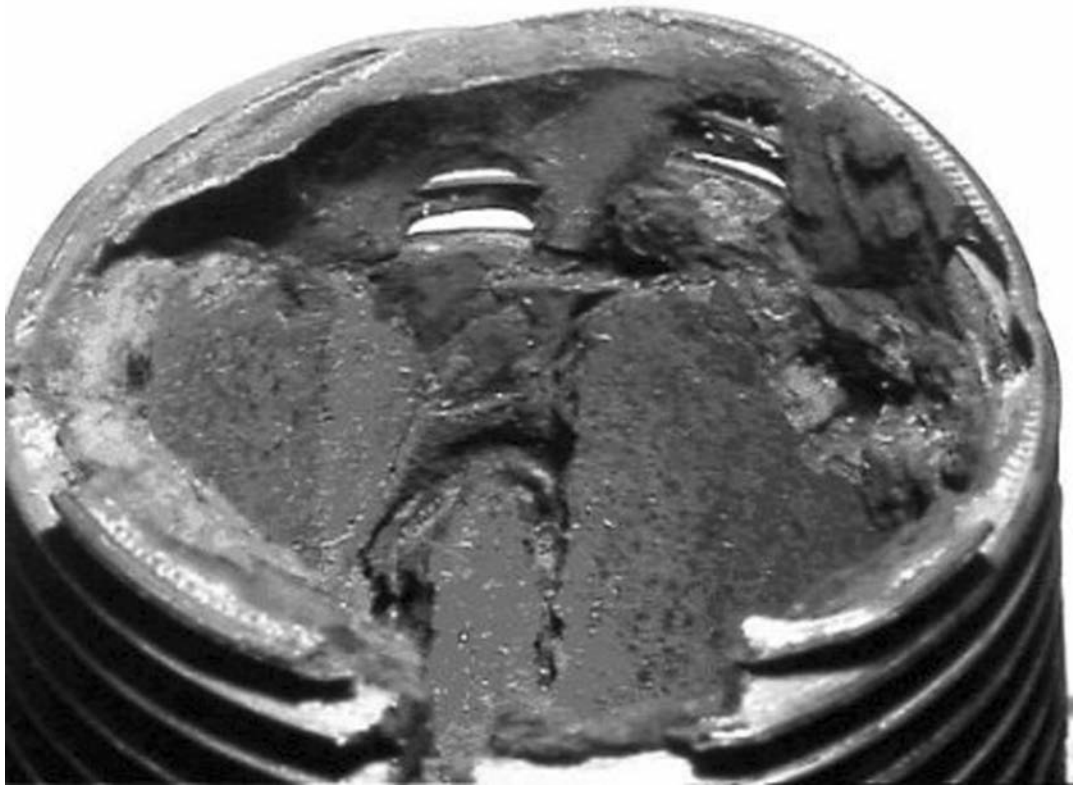
Fig. 4-43—CO 2 corrosion of CS pipe nipple in CO 2 contaminated water.
