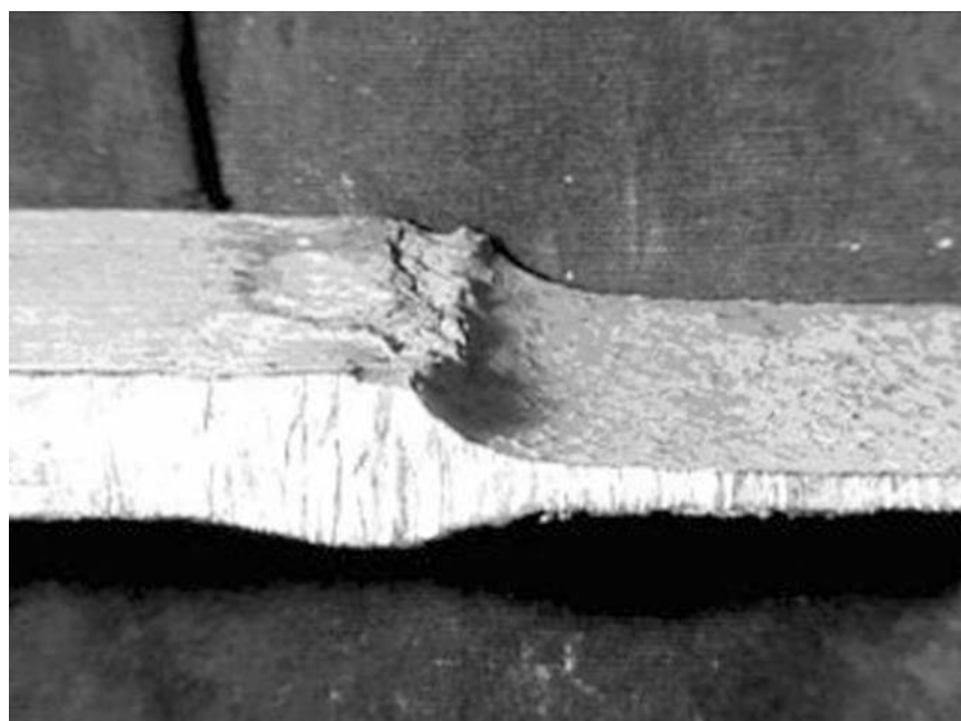
Fig. 5-5—Cross-section of a carbon steel pipe showing preferential corrosion of the pipe with high residual element content on the right (%Cu + %Ni + %Cr), as compared to the low residual pipe section to the left of the weld.
