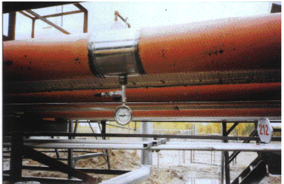
Figure 23: Typical Beta Foil Installation
