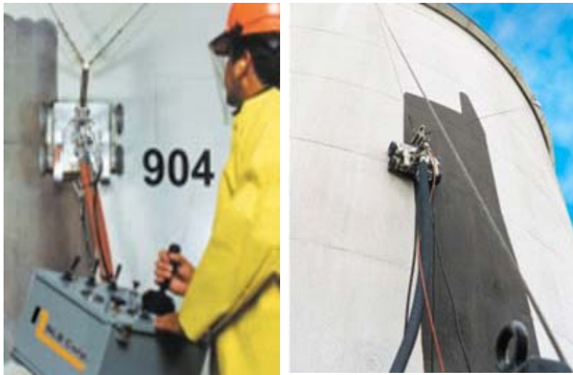
Figure 5.4 Robotic Waterjetting Unit
