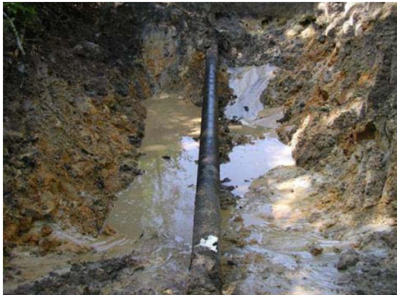
Figure 13.8 Excavation at DG-ICDA Site 4
