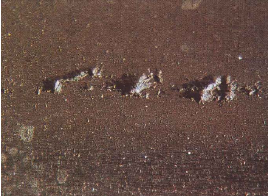
Figure 9.1 Shallow Aligned Gouges on the Internal Surface of a Pipe
