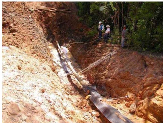
Figure 13.4 Excavation at DG-ICDA Site 2
