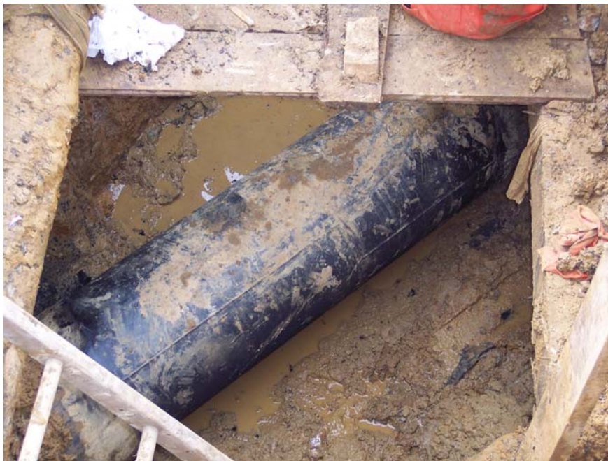
Figure 13.18 Damaged Coating
