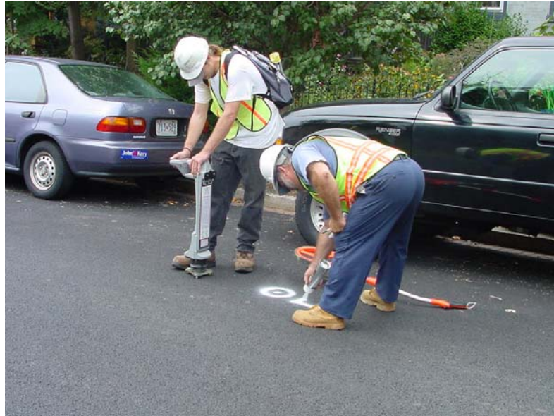
Figure 13.14 Marking Hole Location for Indirect Inspection
