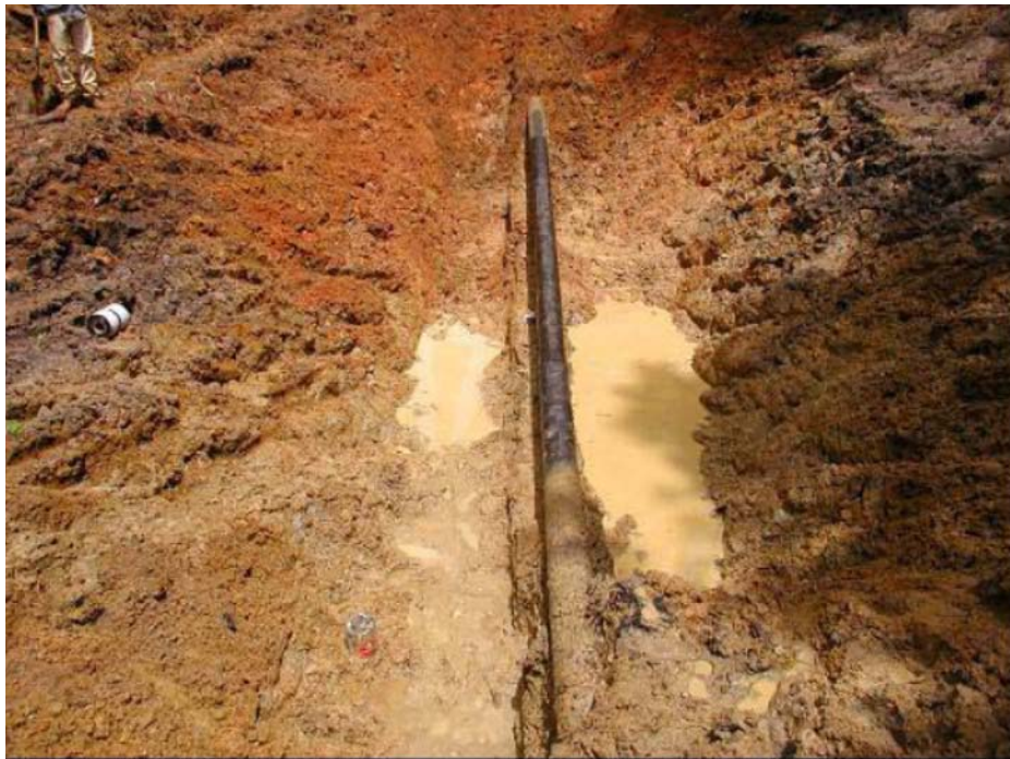
Figure 13.10 Excavation at DG-ICDA Site 5
