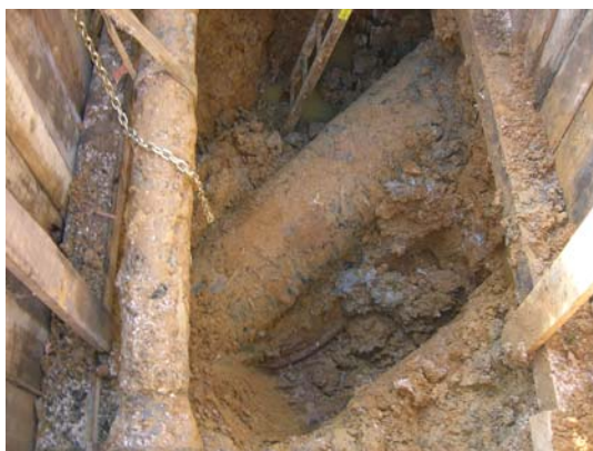
Figure 13.16 Foreign Pipelines in Close Proximity
