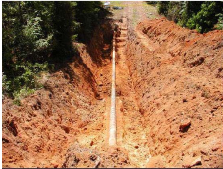
Figure 13.6 Excavation at DG-ICDA Site 3
