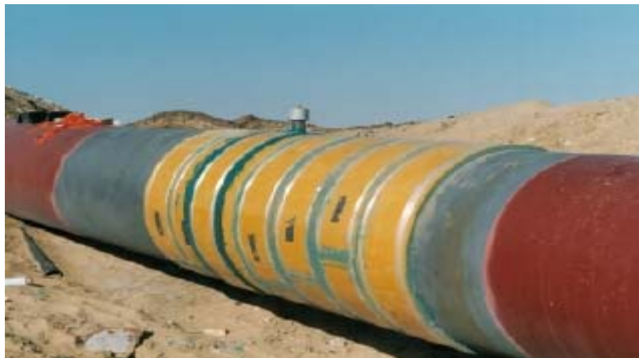
Figure 2.31 Composite Wrap
