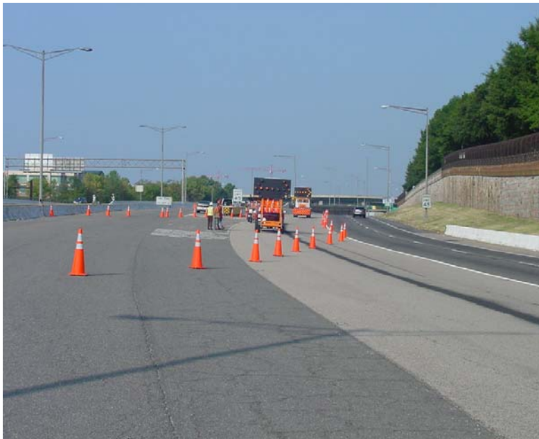
Figure 13.13 Traffic Control for Indirect Inspections
