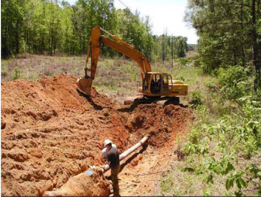
Figure 13.2 Excavation at DG-ICDA Site 1
