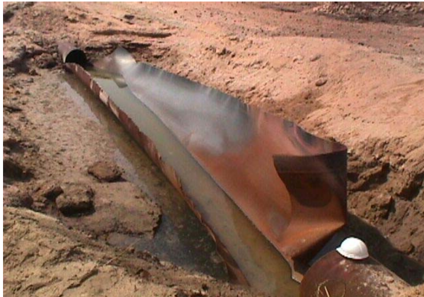
Figure 2.23 SCC-Induced Gas Pipeline Rupture (1999) Accompanied With Rapid Crack Propagation (RCP) (32" O.D. x 0.25 w.t. API 5L Grade X60; MAOP=434 psi)
