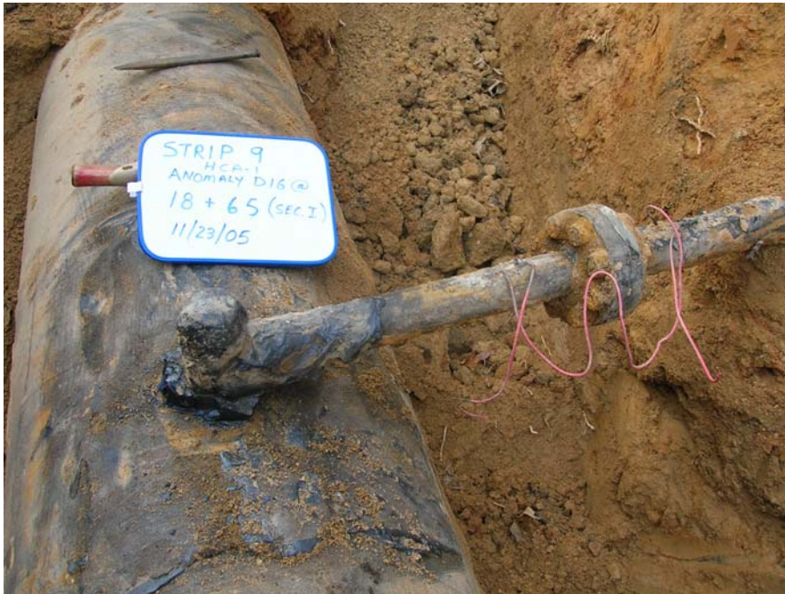
Figure 13.17 Two Inch Service Connection
