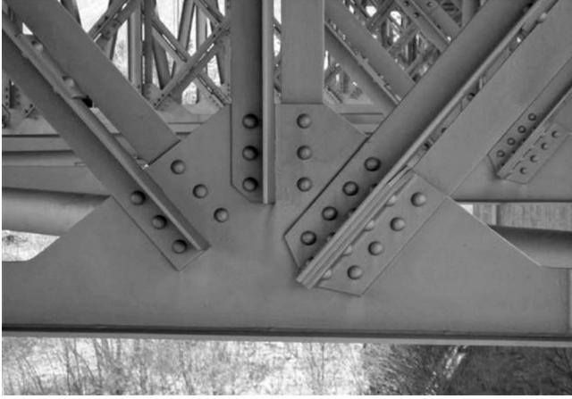
FIGURE 13.3 Detail from Rombak Bridge. No corrosion can be found almost 40 years after application of the original coating. Even at lap joints like this, where the coating is unable to penetrate into the crevice between the overlapping steel parts, there is no sign of corrosion. (Photo: Reidar Klinge, NPRA.)
