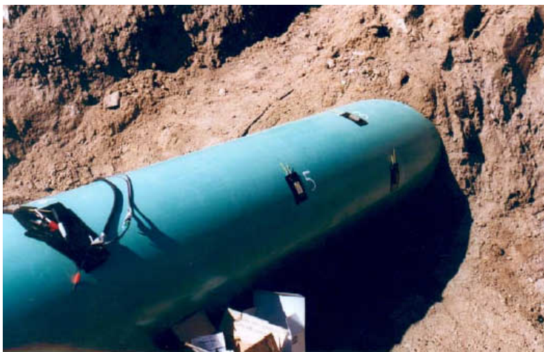
Figure 7-11. Soft cells and a calibration cell attached to coated pipe surface at Site #1 for EIS measurements [King et al., 2002].
