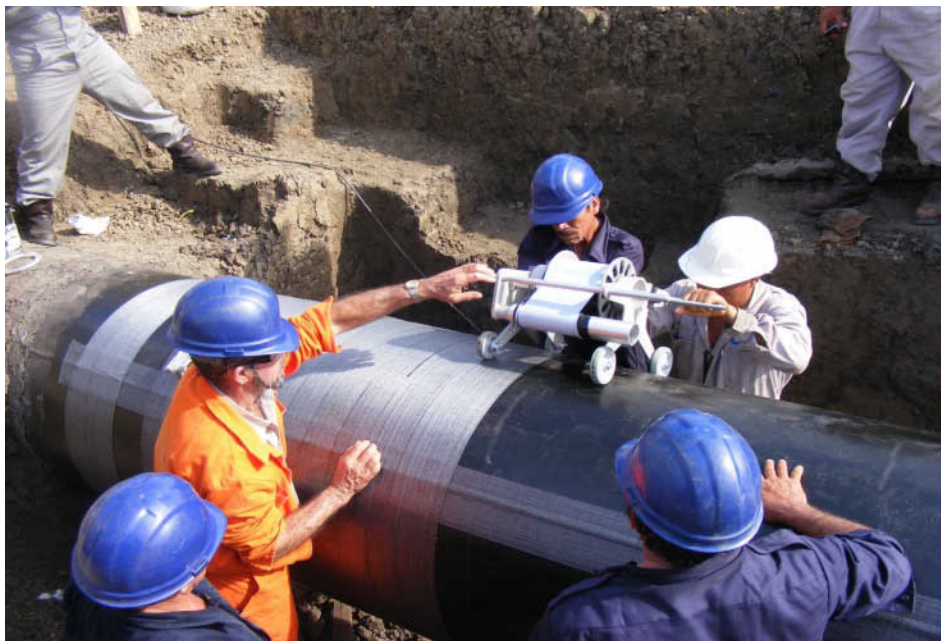
Figure 8-3. Mesh- backed tape being applied with a hand wrapster.
