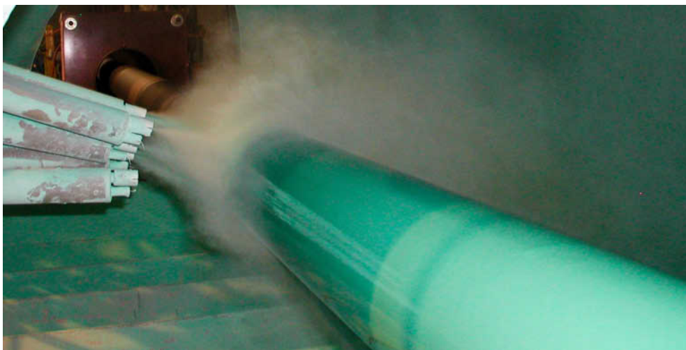
Figure 8-1. Electrostatic spray process for FBE on heated pipe.
