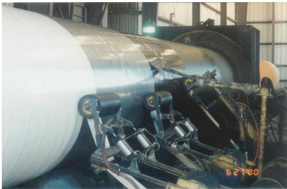
Figure 8-4. Plant application of three layers of solid film-backed tape on water pipe.
