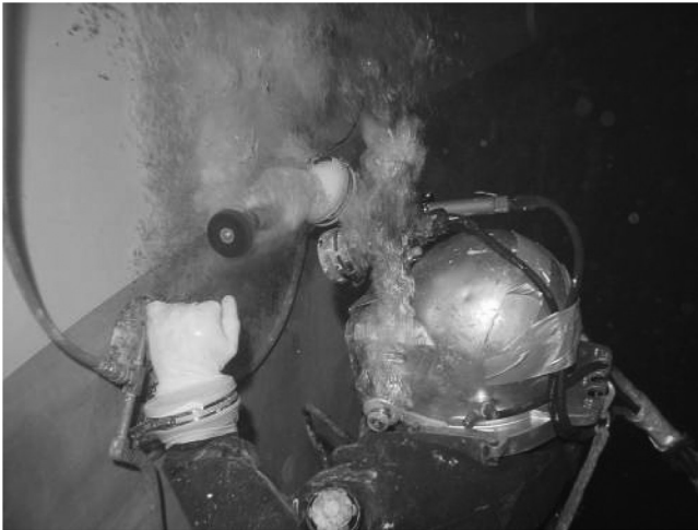
FIG. 13.6 Underwater surface preparation (courtesy of Underwater Engineering Services, Inc.).
