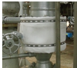
Valve with and without the installed FIRESAFE Fire Protector.
