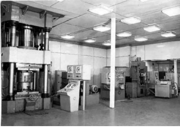
Fig. 10. Pilot production shop for forging under Superplasticity conditions: 1 – hydraulic press, 2 – universal heating device, 3 – electric furnace, 4 – thermostat for regulated cooling of parts.
