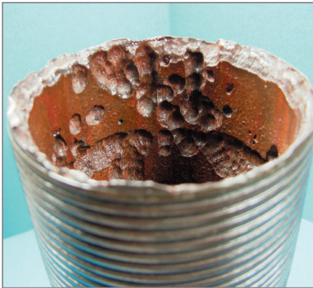
Example of CO 2 corrosion of Carbon Steel OCTG pipe
