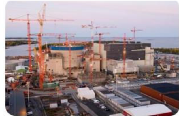
Olkiluoto 3, Construction site
