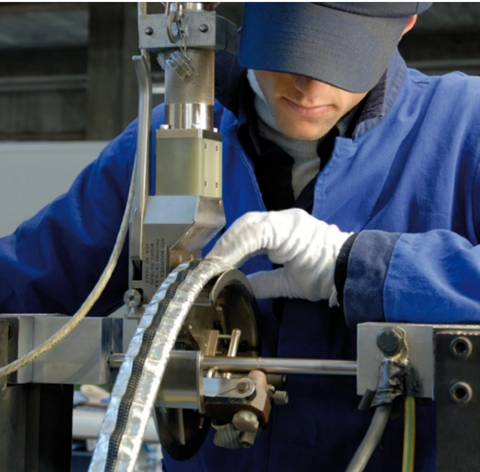
Welding operation at umbilical line
