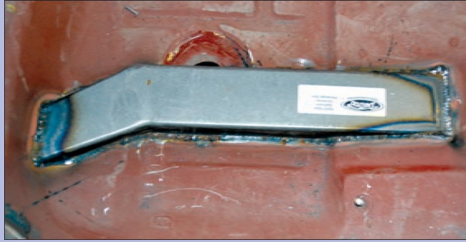
Fig. 6.107. This subframe connector was MIG welded to the early Camaro front and rear subframes but ties into the unibody floor. MIG welds were used to join it to the floor around the circumference.
