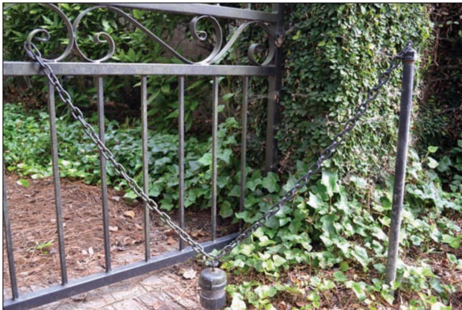
Fig. 6.87. To close the gate an old colonial system was used: a cannon ball and chain. Gravity pulls the gate closed. A simulated cannon ball was made from a pipe nipple and caps, which allowed adding weight so the exact amount of metal scrap could be added to the center cavity and adjusted for proper closure without excessive force.
