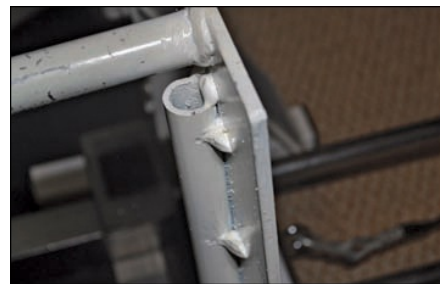
Fig. 6.126. A 1-inch-diameter pipe was welded to the back of the upper foot support to provide the needed stiffness. Although small gussets could have been used, a total of 10 were made from weld metal using overlapping tack welds. This provided the strength needed for what is equivalent to a 715-pound angled leg press machine employing weight plates found in a typical gym.
