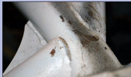
Fig. 6.116. This is a close-up view of the welds on the top of the driver-side roll cage. They were subjected to the impact as the car flipped eight times down the track. All welds held perfectly; there are no cracks. Note the small gusset used at one of the intersections.
