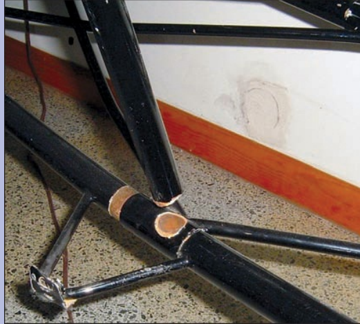
Fig. 4.76. This older chrome-moly dragster frame obviously failed during a crash. The weld is very small and broke with no deformation. With the proper size, shape, and quality of weld, the tubes should have deformed before this failure occurred.
