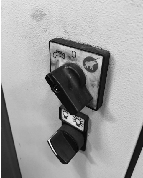
Figure I.5. Icons on the emergency wash. Note the elephant to indicate a spray.
