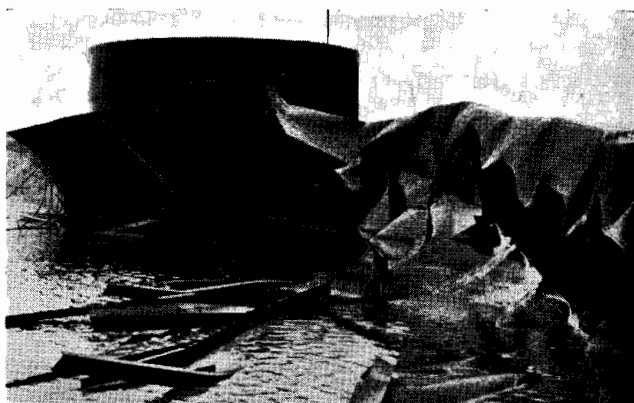
FIG. 43—One of Two Cone-Roof Storage Tanks That Failed During Hydrostatic Testing. Ambient temperature was +40 F.
