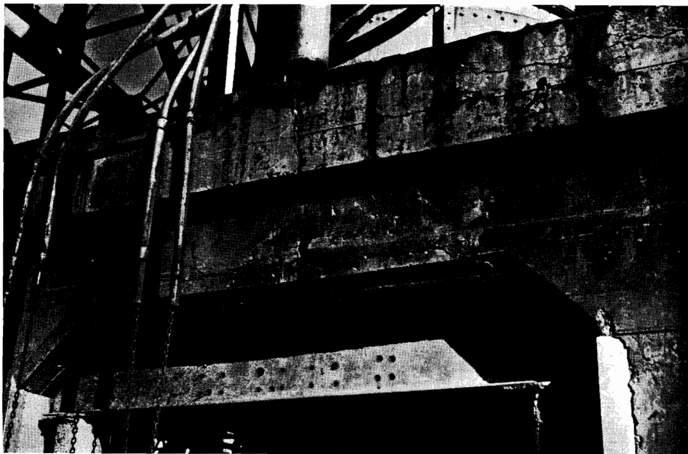
FIG. 54—Deterioration of the Concrete Foundation Pedestal in One of the Areas of Maximum Stress.
