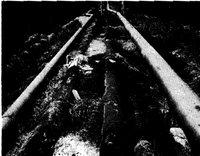
FIG. 27—Half-Buried Lines Such as These Suffer Severe Corrosion of the Type Shown in Fig. 28.
