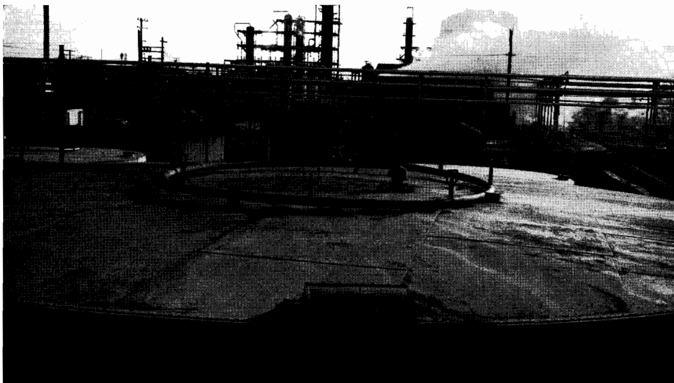
FIG. 14—Severe Corrosion of Cone-Roof Tank Roof.
