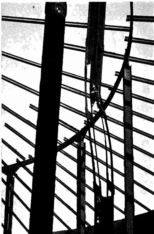
FIG. 15—Severe Vapor-Space Corrosion of Cone-Roof Tank Column.
