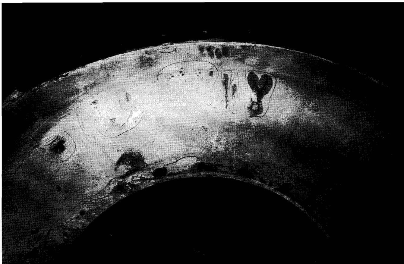
FIG. 32—Intergranular Corrosion in an 18 Chromium-8 Nickel Steel Pressure Vessel Head.
