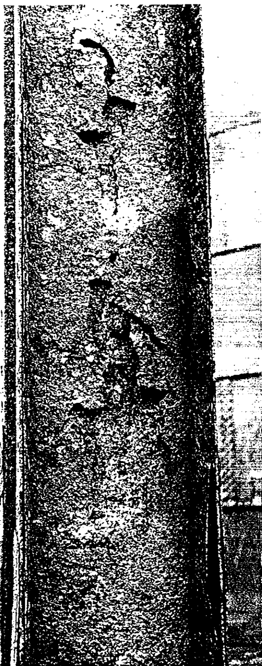
FIG. 17—Close-up of Corrosion of the Column Shown in Fig. 16.
