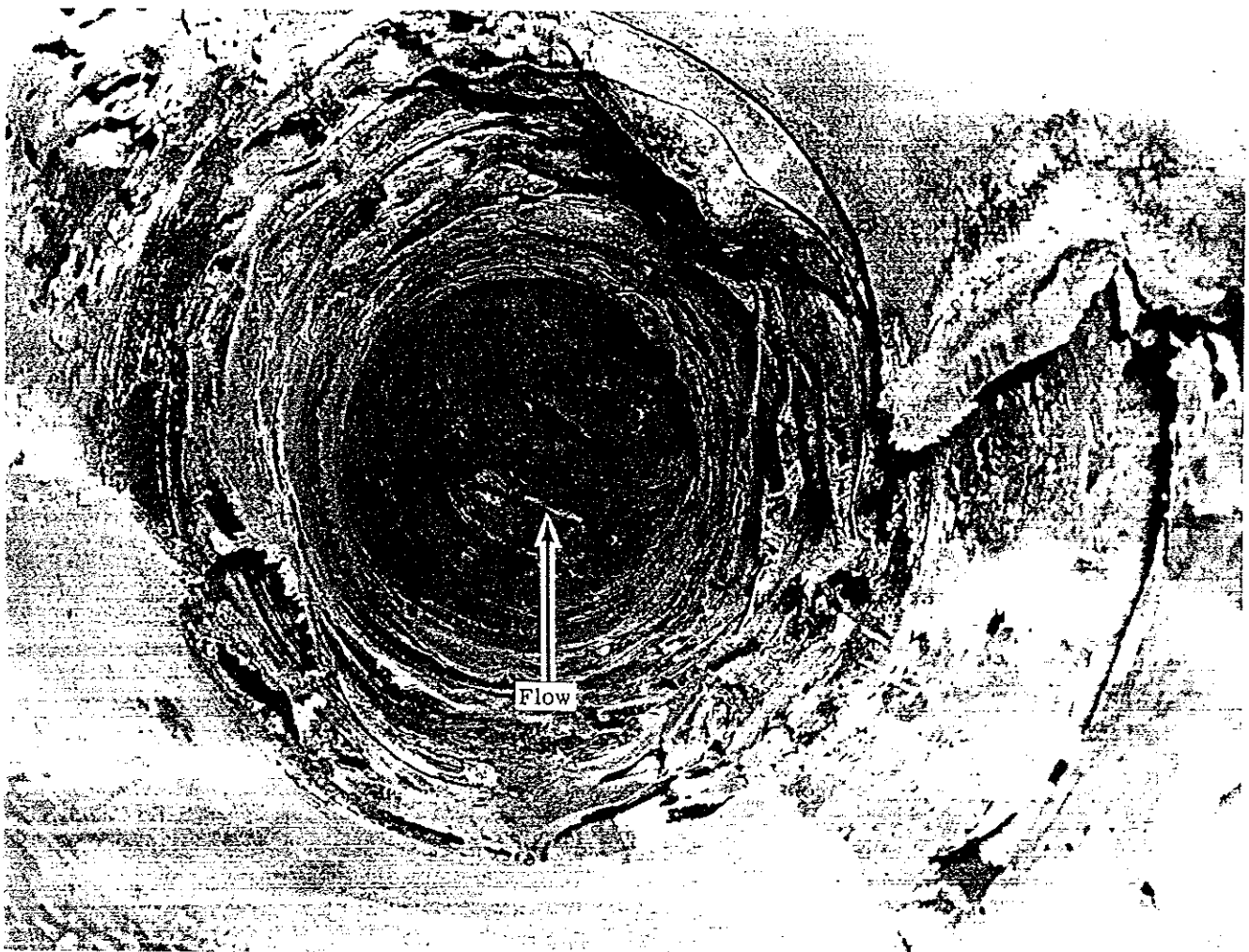
FIG. 38—Deterioration of Liner in Flue-Gas Line on a Catalytic Cracking Unit.
