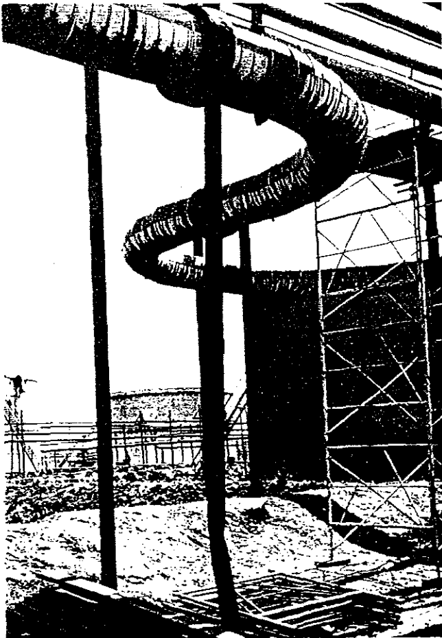
FIG. 49—Overloaded Pipe Support.
