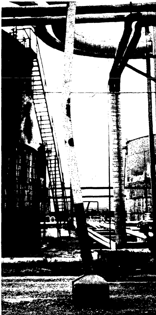
FIG. 56—Pipe Support Column Damaged by Motorized Equipment.
