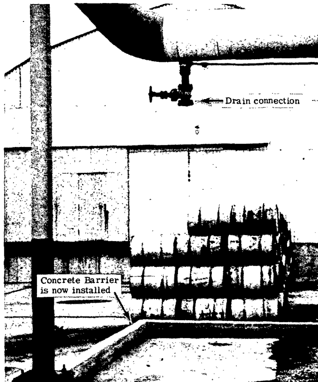
FIG. 57—Drain Connection on High-Pressure Steam Line was Broken Off When a Truck Used the Space Between the Pipe Support Columns as a "Turnaround Area" for Access to Warehouse Doors.
