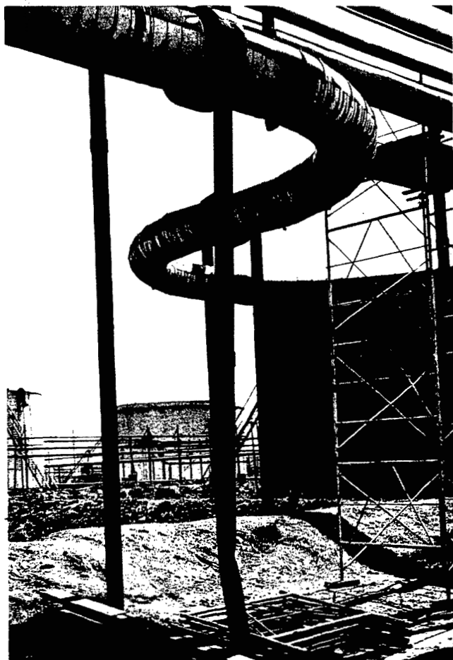
FIG. 49—Overloaded Pipe Support.
