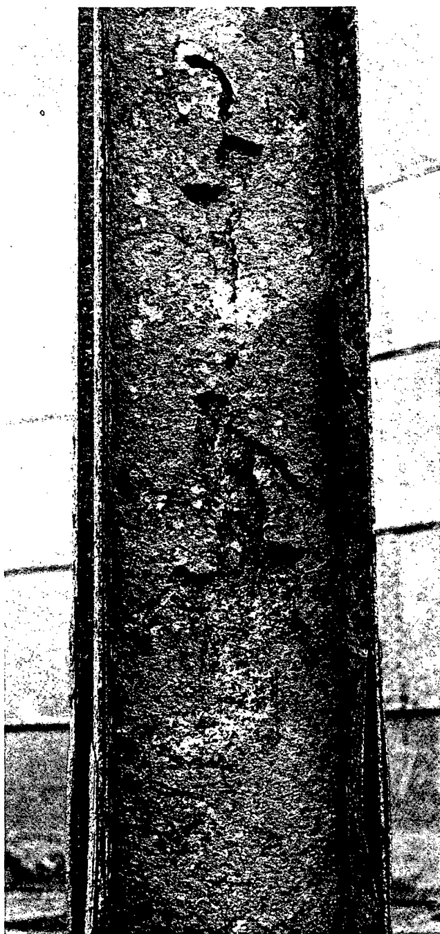
FIG. 17—Close-up of Corrosion of the Column Shown in Fig. 16.
