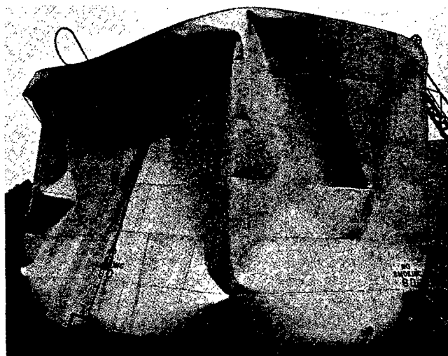
FIG. 45—Collapse of an Atmospheric Storage Tank as a Result of Inadequate Vacuum-Venting Capacity.
