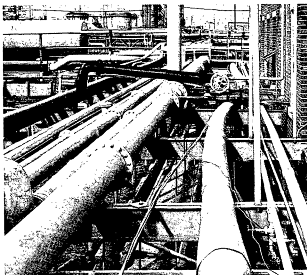
FIG. 55—Wooden Support is Inadequate to Support Overhanging Piping.
