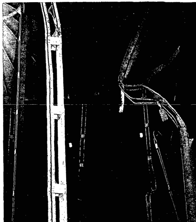
FIG. 53—Tank-Roof Supports Are Overloaded After Corrosion Has Occurred.
