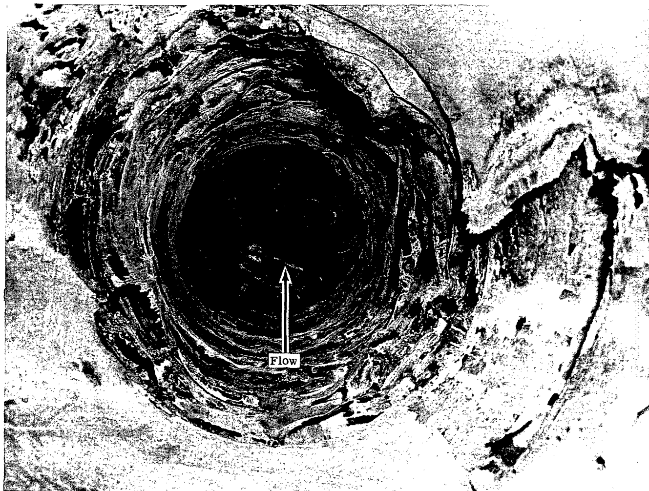
FIG. 38—Deterioration of Liner in Flue-Gas Line on a Catalytic Cracking Unit.
