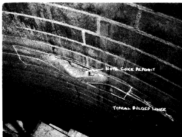
Figure 28—Strip-Lining Deterioration
