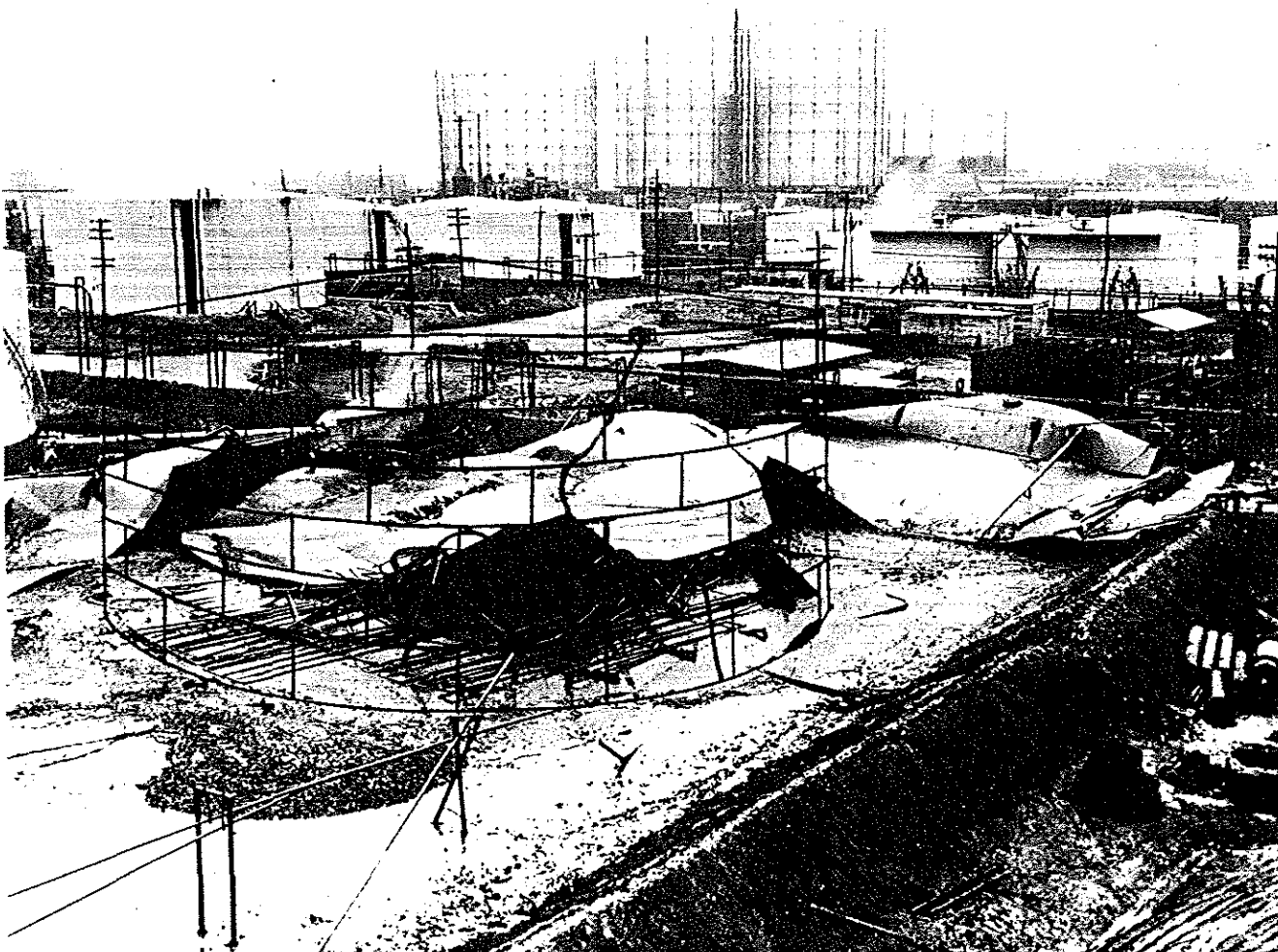
Figure 28—Damage from Instantaneous Failure
