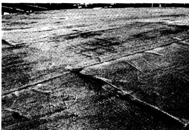
Figure 63—Mastic Roof Coating
