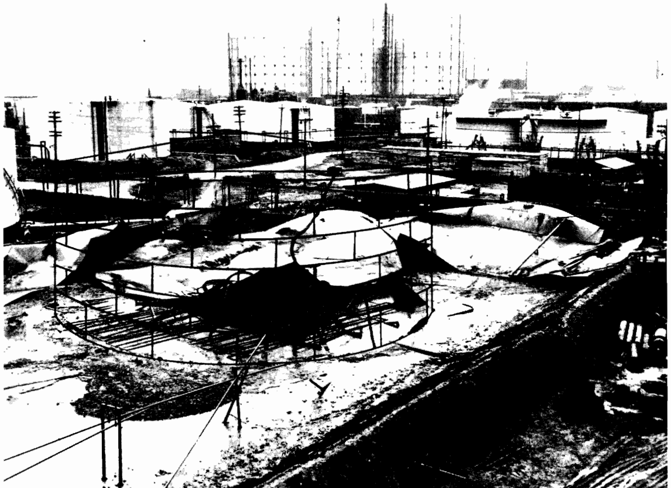
Figure 28—Damage from Instantaneous Failure
