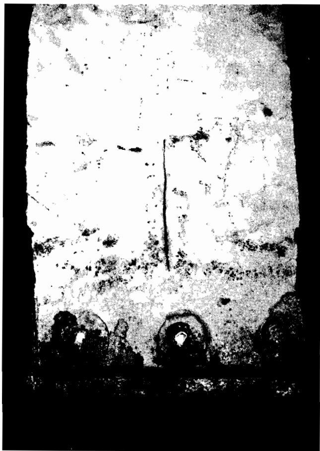
Figure 29—Cracks in Tank Shell Plate
