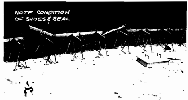
Figure 42—Deterioration of Floating Roof Seal
