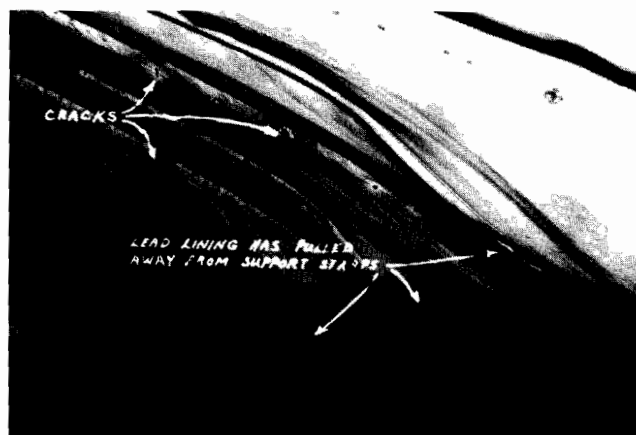
Figure 53—Deterioration of Lead Lining on Roof of Tank Caused by Leaks in Lining
