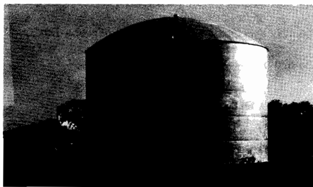
Figure 2—Umbrella-Roof Tank
