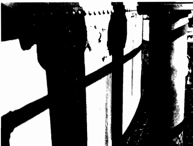
Figure 49—External View of Corrosion-Erosion Completely Through a Tank Shell
