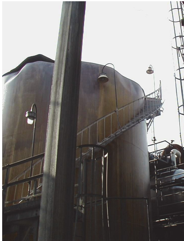
Figure 44—Roof Overpressure
