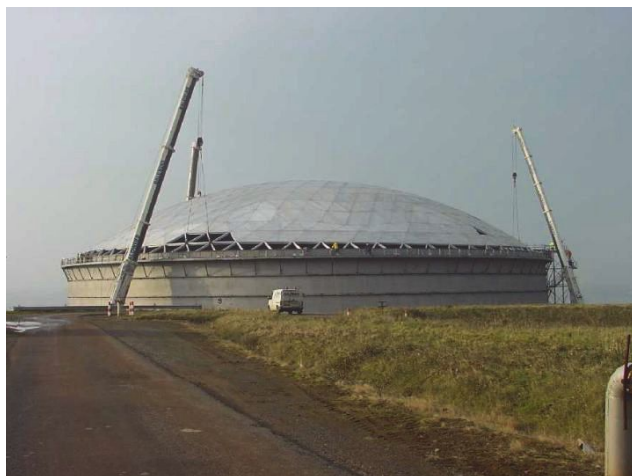
Figure 3—Geodesic Dome Roof Tank
