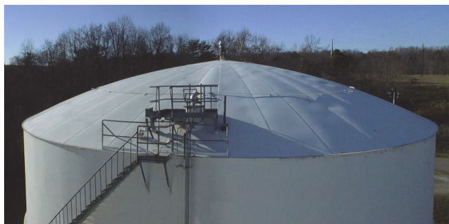
Figure 2—Umbrella Roof Tank
