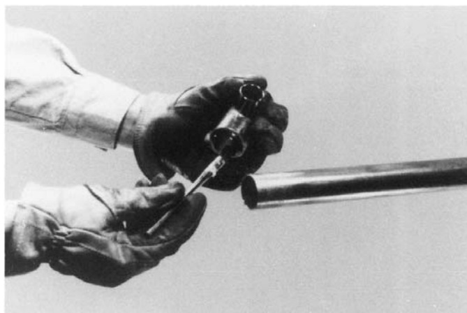
FIG. 11 Fluxing: Fitting
