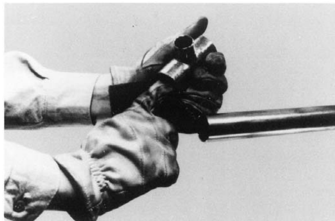
FIG. 8 Cleaning: Abrasive Pad
