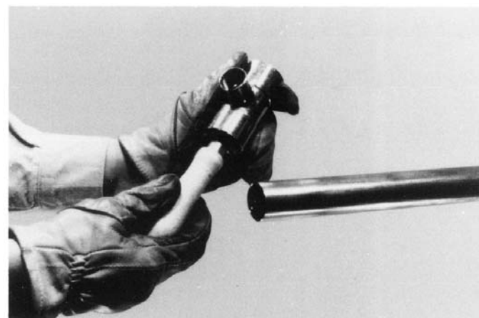
FIG. 9 Cleaning: Fitting Brush
