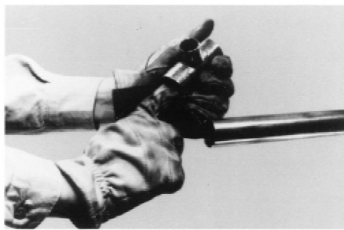
FIG. 8 Cleaning: Abrasive Pad
