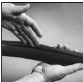
FIG. 3 Apply Unslit Insulation to Straight Pipe
