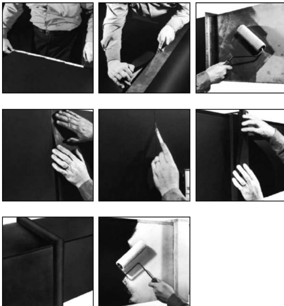
FIG. 13 Duct Covering
