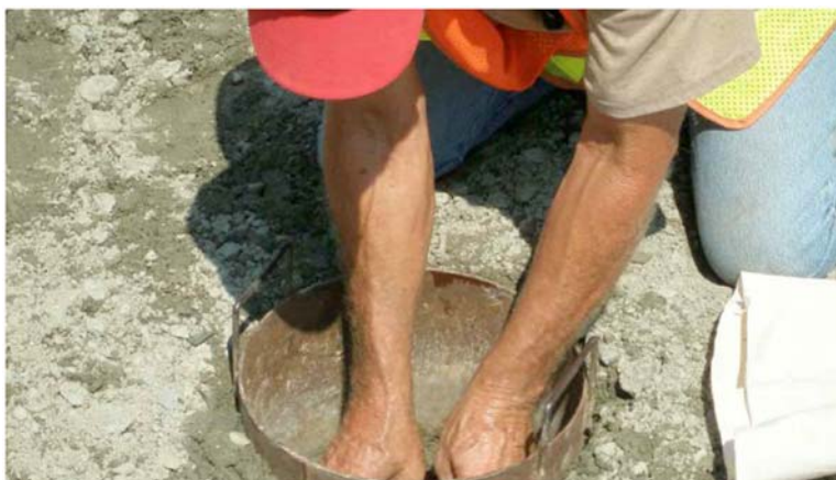
FIG. 5 Proper Use of Metal Template For Sampling Mixed Coarse and Fine Aggregate From Roadway Grade
