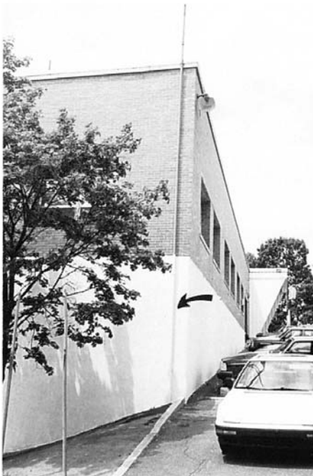
FIG. X1.8 Single Tall Vent Pipe (Arrow) for Underground Storage Tank on Side of Building
