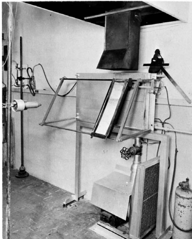
FIG. X2.1 Historic Photograph of Radiant Panel Flame Test Equipment
