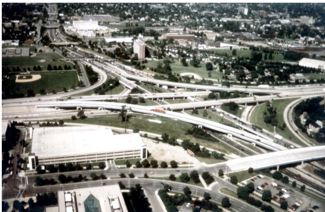
FIG. X2.1 Aerial View of I-94 Interchange
