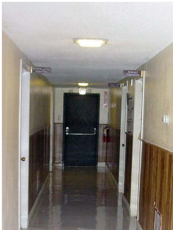
(a) Hallway Ceiling Plaster
