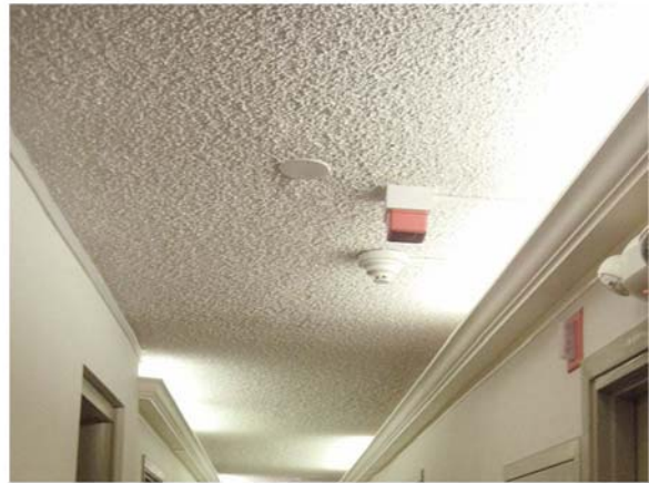
(e) Hallway Ceiling Plaster C5
