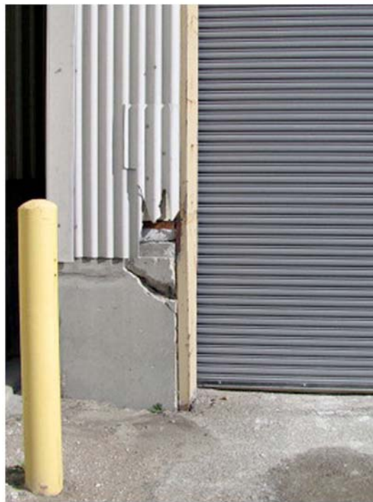
(k) Corrugated Cement Siding W2
