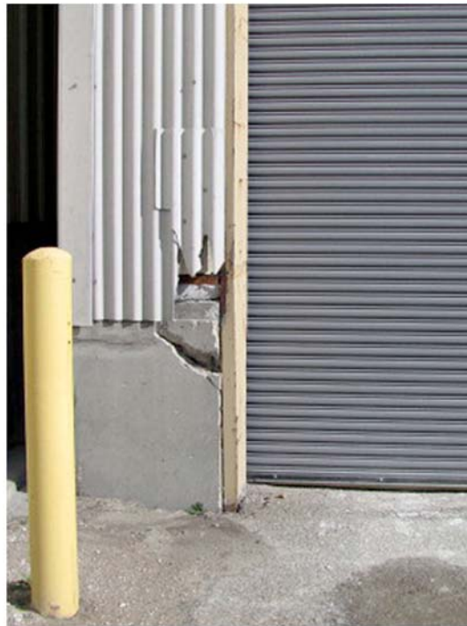
(k) Corrugated Cement Siding W2
