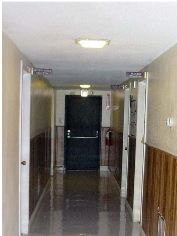
(a) Hallway Ceiling Plaster
