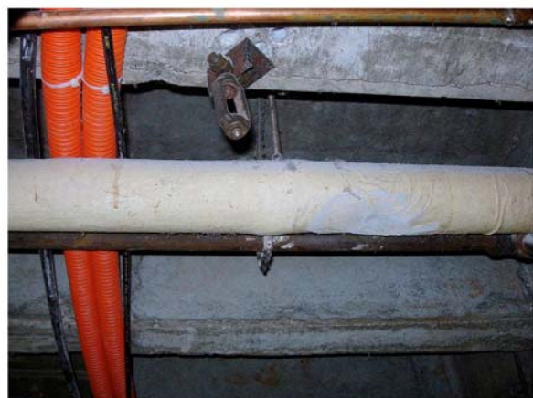
(f) Mechanical Room Pipe hanger P1
