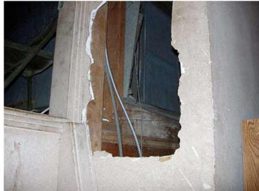
(j) Hallway Wallboard W1
