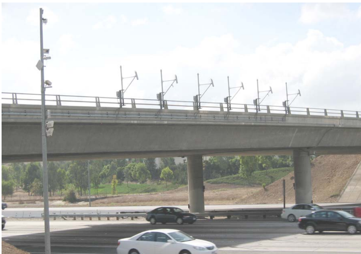
FIG. X2.1 Over-Lane Video Cameras and One of Two Roadside Sensor-Mounting Poles
