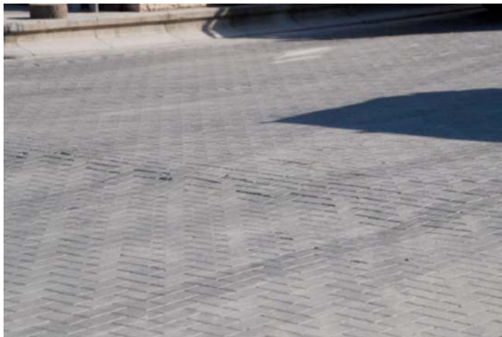
FIG. X1.16 Low Severity Heave
