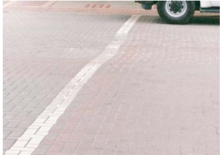
FIG. X1.5 Medium Severity Depression
