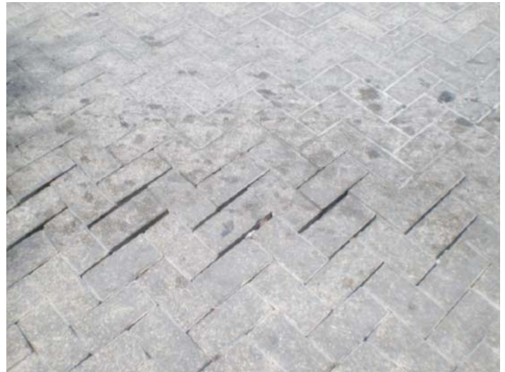
FIG. X1.12 High Severity Excessive Joint Width (greater than ½ in. (13 mm))
