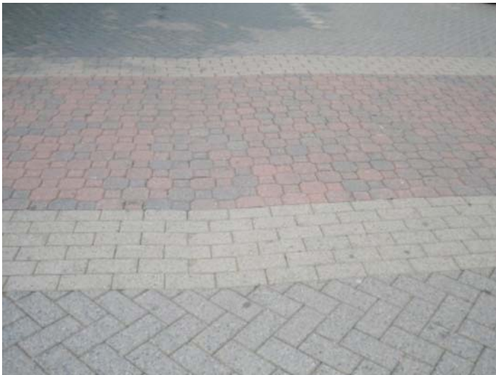
FIG. X1.4 Low Severity Depression
