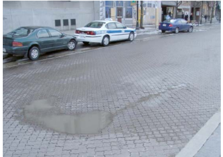
FIG. X1.6 High Severity Depression
