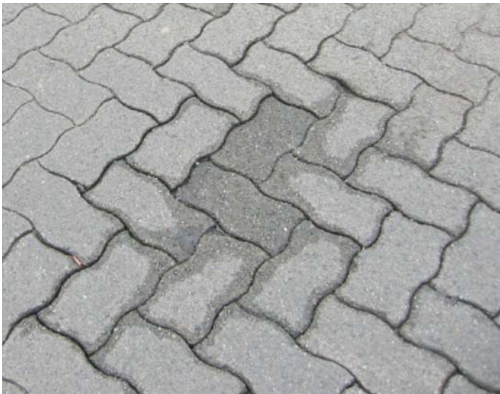
FIG. X1.10 Low Severity Excessive Joint Width (Approximately ¼ in. (6 mm) wide and performing well)
