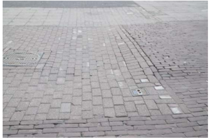
FIG. X1.17 Medium Severity Heave
