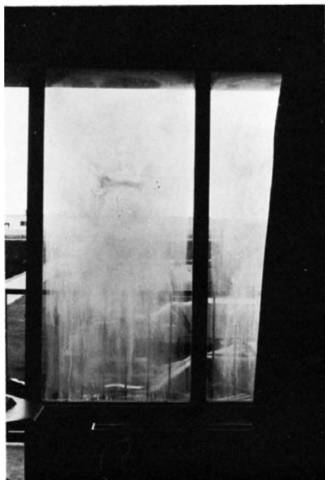
(b) Scummed and Stained Interior Glass Surface
