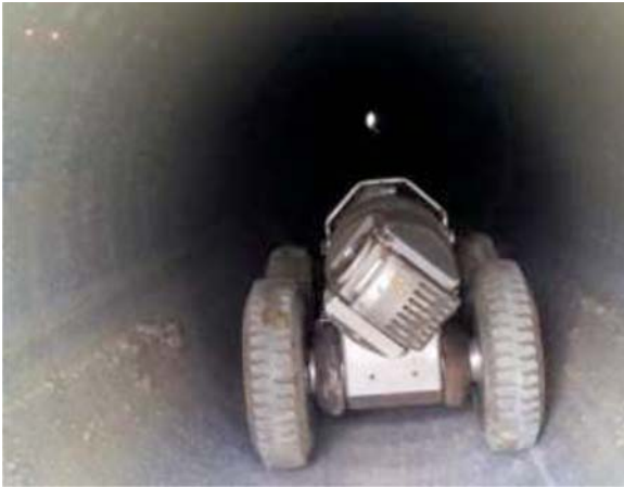
FIG. 1 CCTV—Rotating Laser Profile Camera in Pipe
