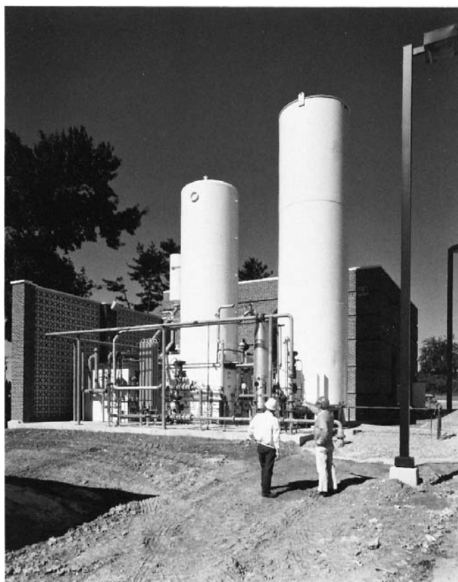
FIG. 1 High-volume Oxygen Users Buy the Gas in Bulk, Storing It in an Adjacent Facility
