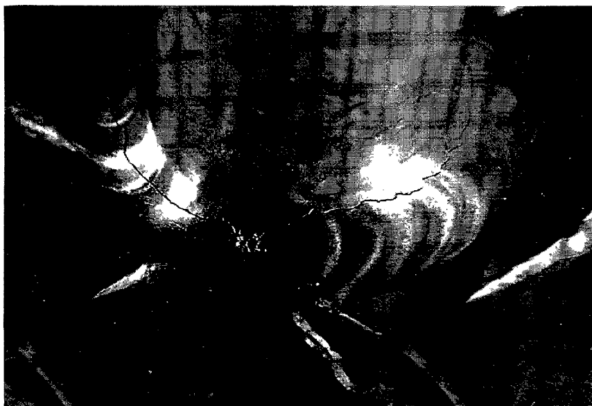
LONGITUDINAL CRACK PROPAGATING FROM CRATER CRACK
