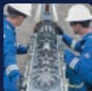
ONSTREAM INLINE PIPE INSPECTION
