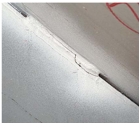
Figure 9 Crack found using Magnetic Particle Inspection
