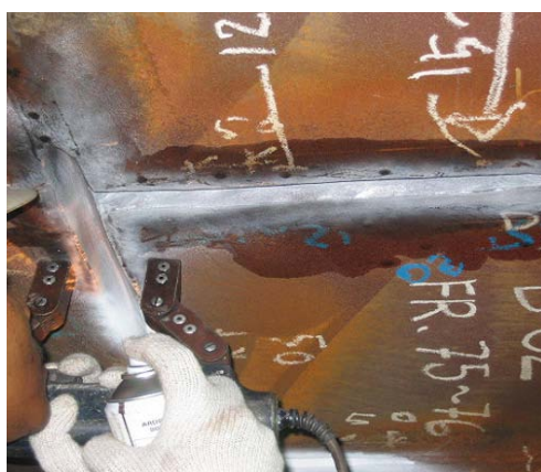
Figure 8 Magnetic Particle Inspection using a yolk
