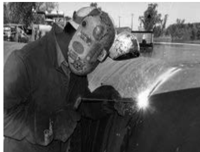
Examples of the MMA welding process.
