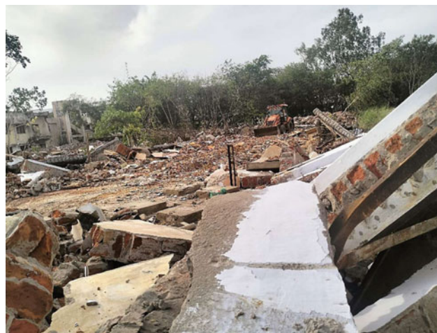
Fig. 1 CDW from 30 years old university building
