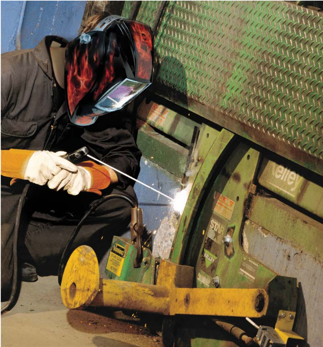
Illustration 5-5 Shielded Metal Arc Welding is widely used for Maintenance and Repair
