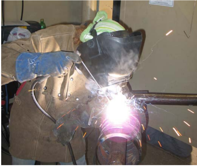
Illustration 14-2 – Shielded Metal Arc Welding Pipe
